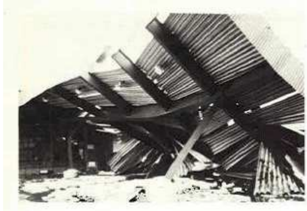
Figure 2.3: Canopies built in 1975. The primary beam is left unbraced on the compressed side above the supports (columns). The beam probably failed due to lateral torsional buckling. It appears as though thereafter the columns buckled at their tops as a consequence of the large deformations that occurred. (Johannesson et al. [9])
